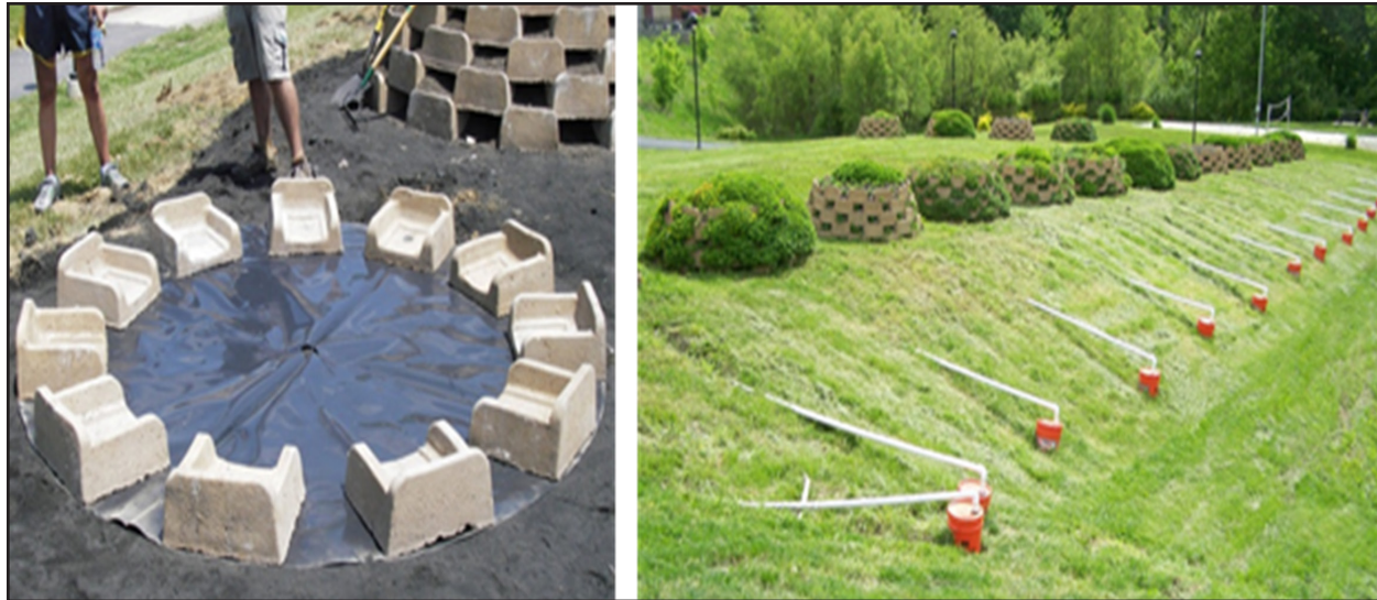
Fig. 1. Green retaining wall design. (a) Each green retaining wall system was designed with an impervious base layer (foreground). Blocks are arranged in 5 staggered tiers (background). (b) Each system was also fitted with 20.4 L stormwater collection units (June 2010).
